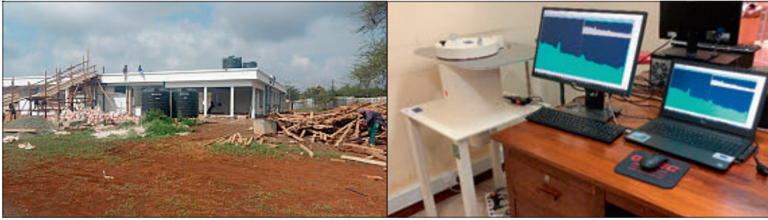
Figure 18. Infrastructure and capabilities – new facilities in advanced construction with new equipment at Tanzania Atomic Energy Commission (TAEC) Arusha, August 2018
