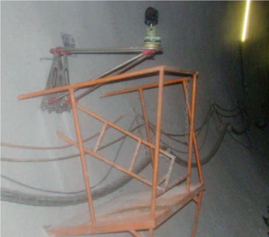
Fig. 7: Measurement console with footing platform.
