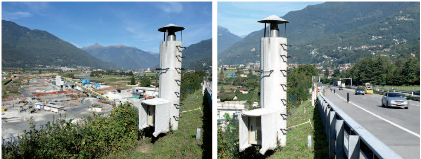
Fig. 2: Survey pillar: Automatic monitoring along the A2 motorway – the monitoring system detects movements to a predetermined sensitivity of 3 mm.
