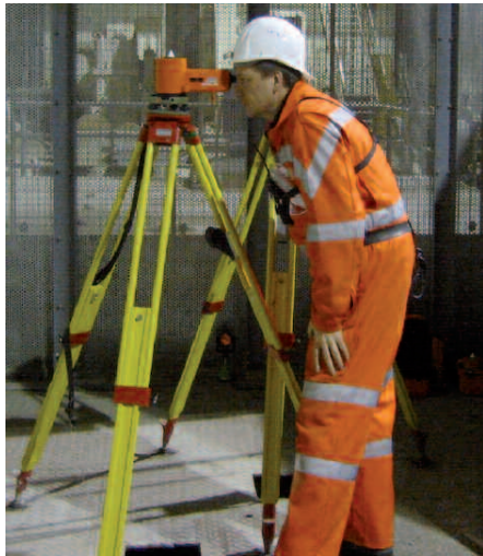
Fig. 4: Nadir plummet at head of shaft.
