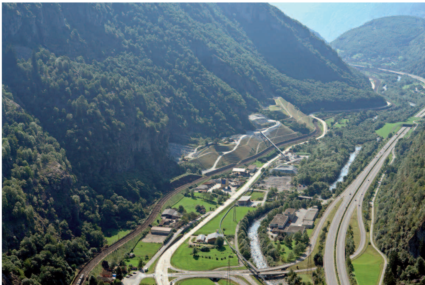
Fig. 3: Overview of landfill site Chiggiogna/Cavienna, south of the Faido access tunnel.
