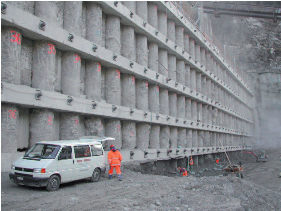
Fig. 2: The approximately 30-m-high drilled pile retaining wall (Photo: Basler & Hofmann).
