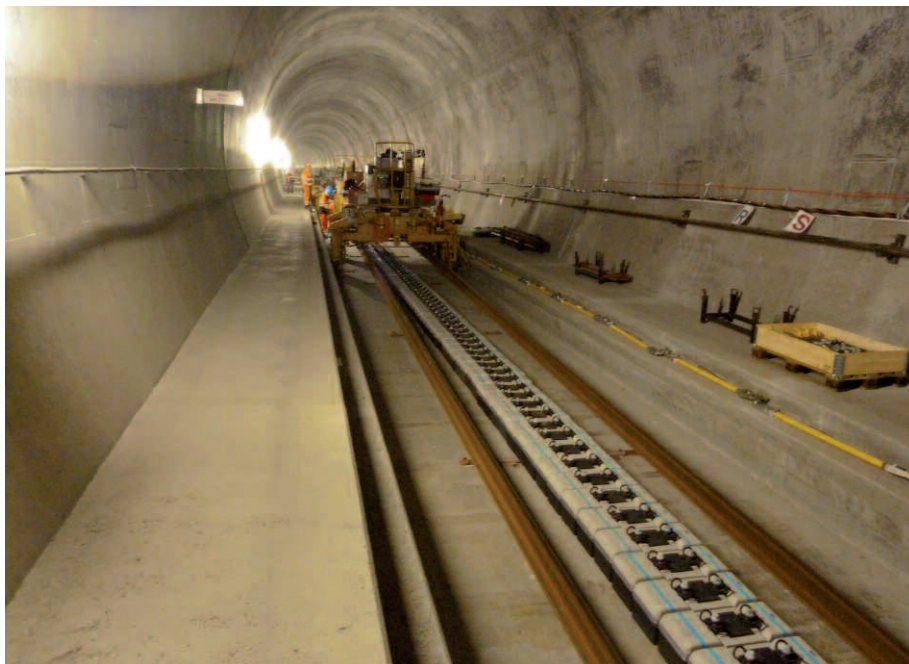
Fig. 4: Track laying in the section Bodio – Faido West.
