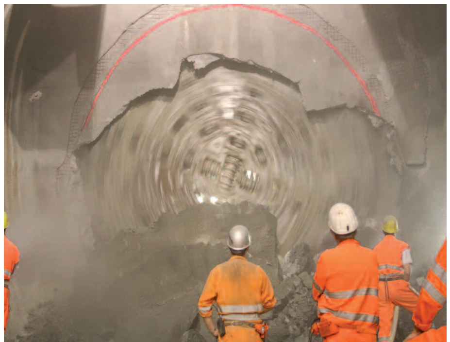
Fig. 12: Boring head of tunnel boring machine at breakthrough.
