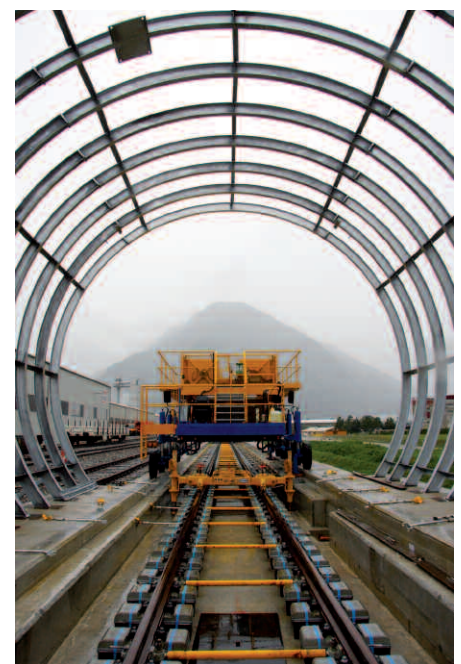
Fig. 1: Training/sample track at the Biasca surface installations site.
