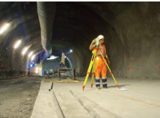
Fig. 2: Staking out in the tunnel.
