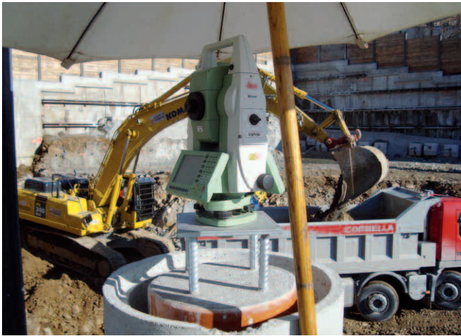
Fig. 5 Monitoring on the building sites.
