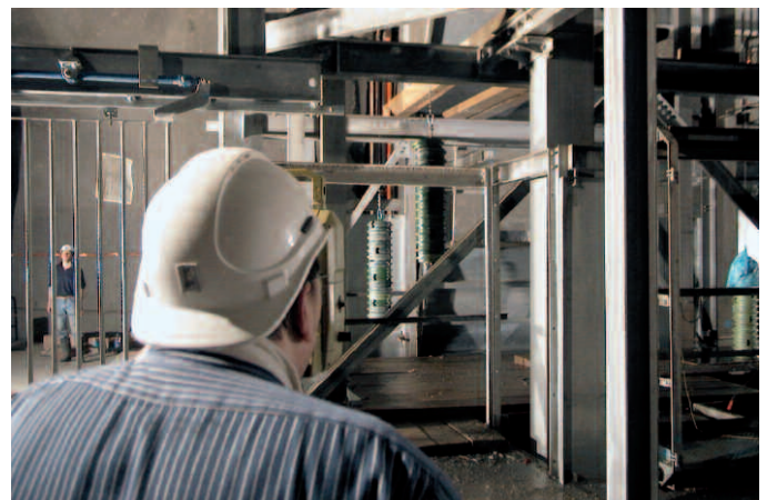
Fig. 7: Plumb bobs with 192 kg loads.
