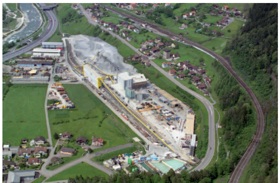
Fig. 2: Overview of external structures and Amsteg section access tunnel.
