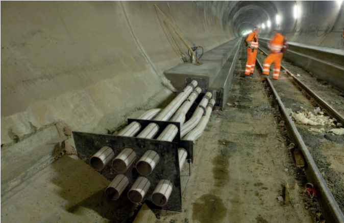
Fig. 8: Construction of the tunnel bench.
