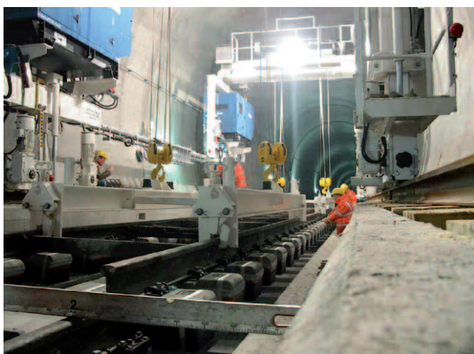
Fig. 4: Installation of the 18 m long track panel.
