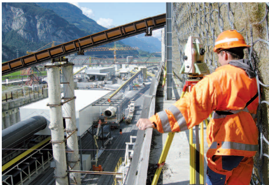
Fig. 4: Geodetic surveying on the drilled pile retaining wall (Photo: Basler & Hofmann).
