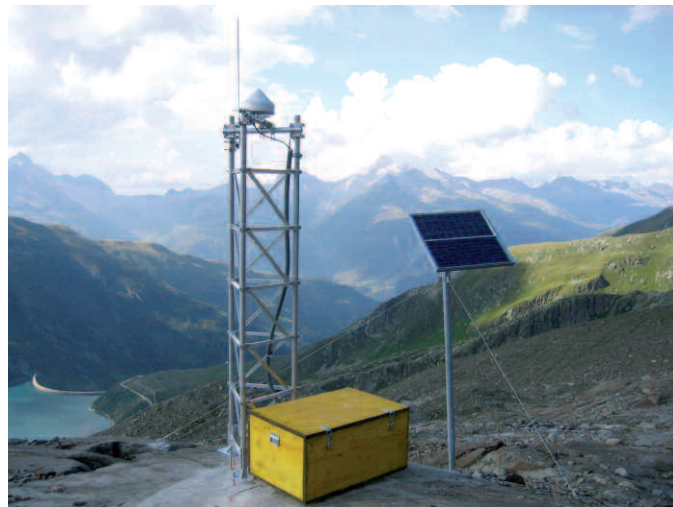
Fig. 6: GPS station above Nalps dam.
