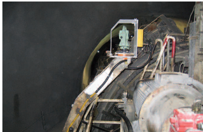
Fig. 6: Divert frame with machine station.
