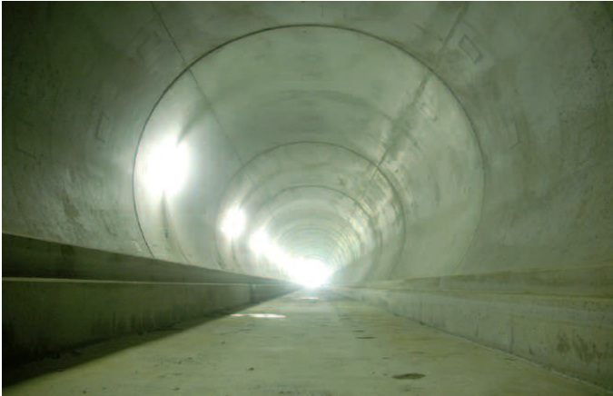
Fig. 9: Concreted, completed tunnel.
