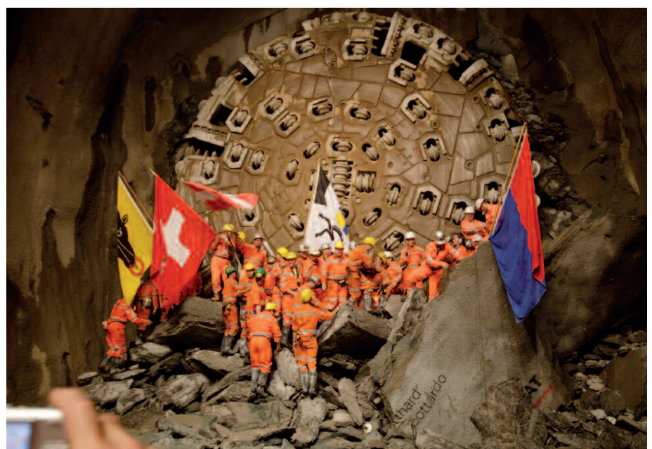
Fig. 3: World record under the Gotthard: on October 15, 2010, the miners celebrated the final breakthrough in the east tube of the Gotthard Base Tunnel.
