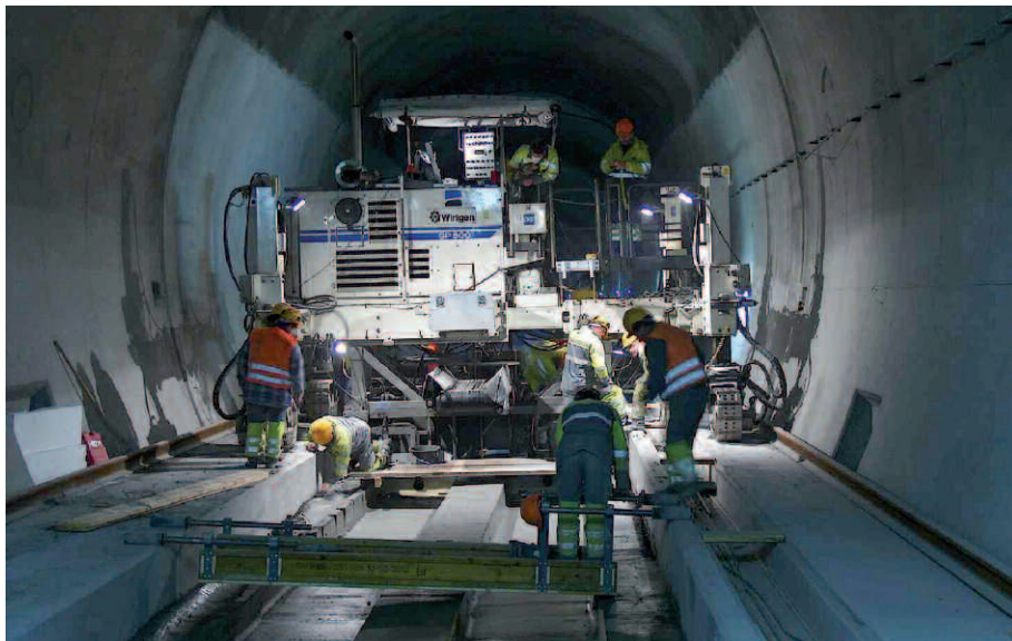
Fig. 8: Installation of the track-supporting slab with the formwork finisher.
