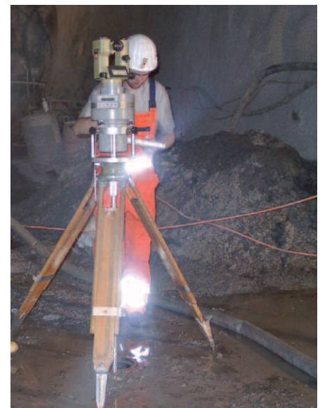
Fig. 8: The gyro-theodolite of the ETH Zürich in action at the Gotthard tunnel.
